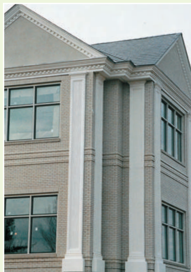
26' Tall Exterior Pilasters
